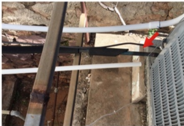
Replace Suction Line Insulation
