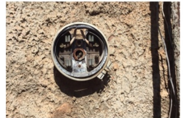
Remove Old Meter Base And Seal Holes
