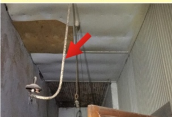
Gas Light, Remove Light And Gas Lines.
