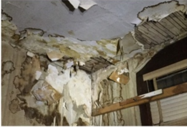
Sever Roof Leak
