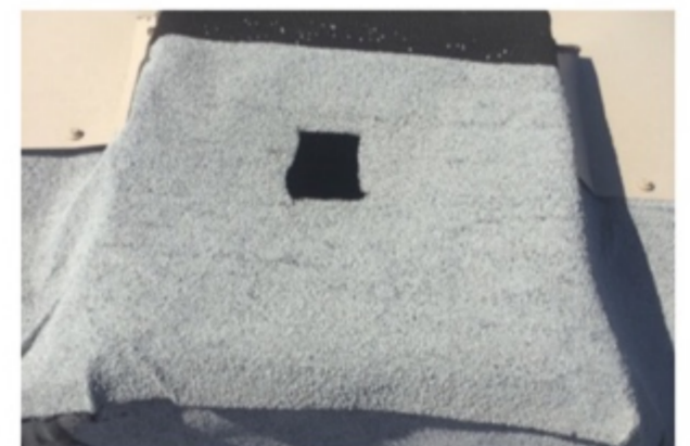
This is the only chimney that is partially covered
