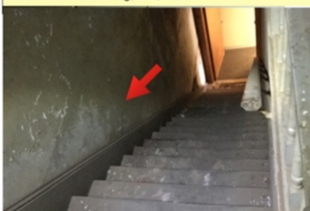
Add Railing On Other Side
