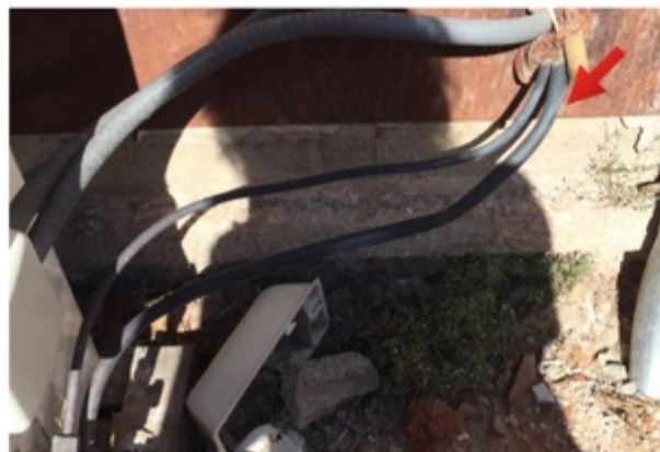
Install Insulation On Both Lines
