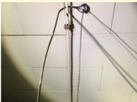
Knob And Tube Wiring, Cut, Remove
