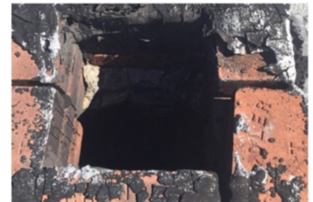
One of the 8 open chimneys
